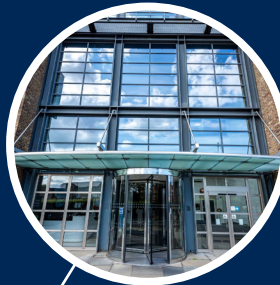
MARTLEY CAPITAL Central Square South Newcastle
